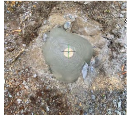
(Capped Post placed within concrete for added stability, NOT A C.M.)
