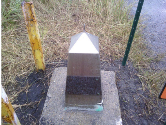
(Restored Steel Sheath of a C.M. monument)
