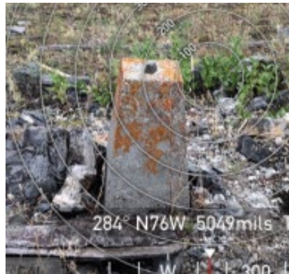
(Unstable Brass Bolt in Concrete, monument was destroyed and replaced with Brass cap at ground level)
