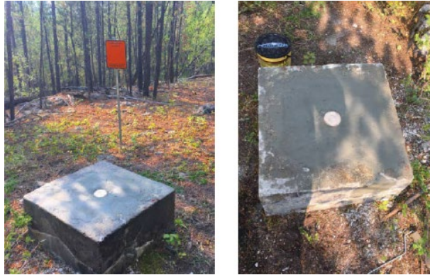
(Brass cap placed in center of restored Concrete Base)
