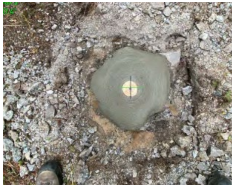
(Capped Post placed within concrete for added stability, NOT A C.M.)
